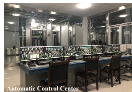
Automatic Control Center
